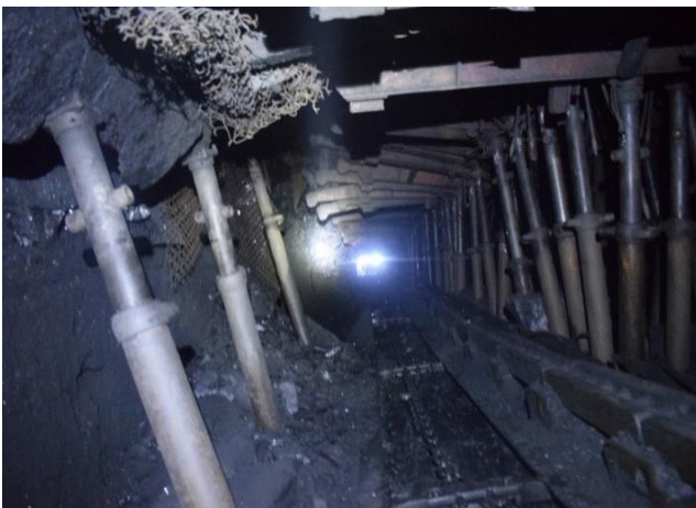
Figure 3. Additional support by hydraulic props at the longwall face I-6-2.
